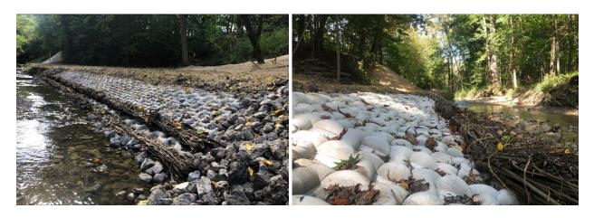
Besides protecting against erosion in a variety of ditch, channel, and embankment settings, VegeMat Fabric Formed Concrete Linings offer the opportunity to revegetate and provide durable, low-maintenance protection long into the future.
