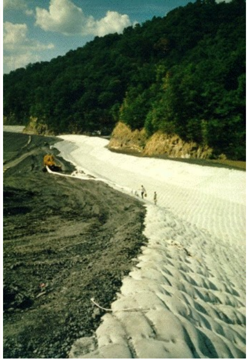
Completed spillway, looking downstream.
