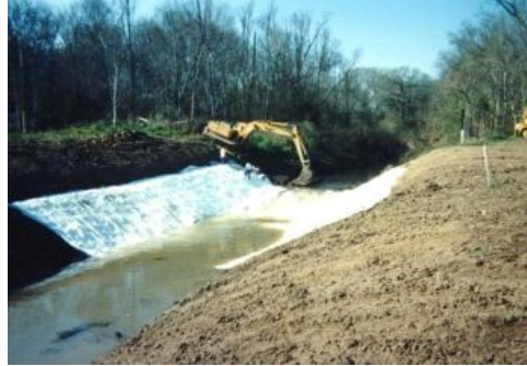
ARMORFORM ABM mat being installed over a restored pipeline crossing
