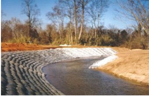
Completed ARMORFORM 6" ABM installation (looking downstream)
