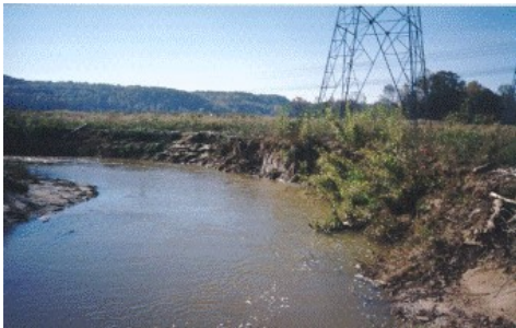
A 500,000 volt electrical tower is dangerously close to the edge of the creek's outer embankment.
